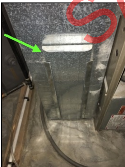
Furnace filter is located here.
