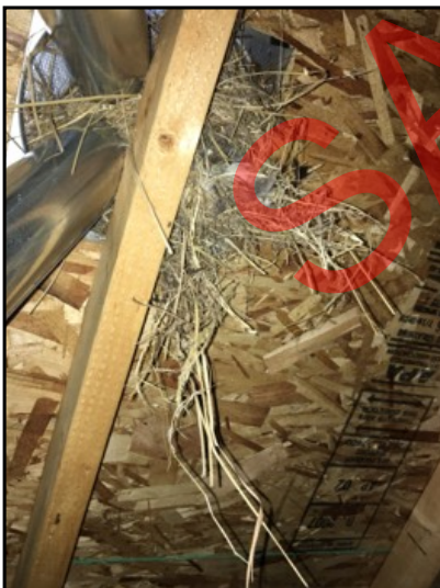
Bird nest in roof vent, screen has been damaged. Recommend repair.
