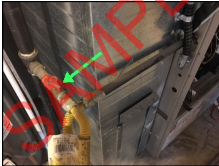
Gas supply shut off valve for the furnace.
