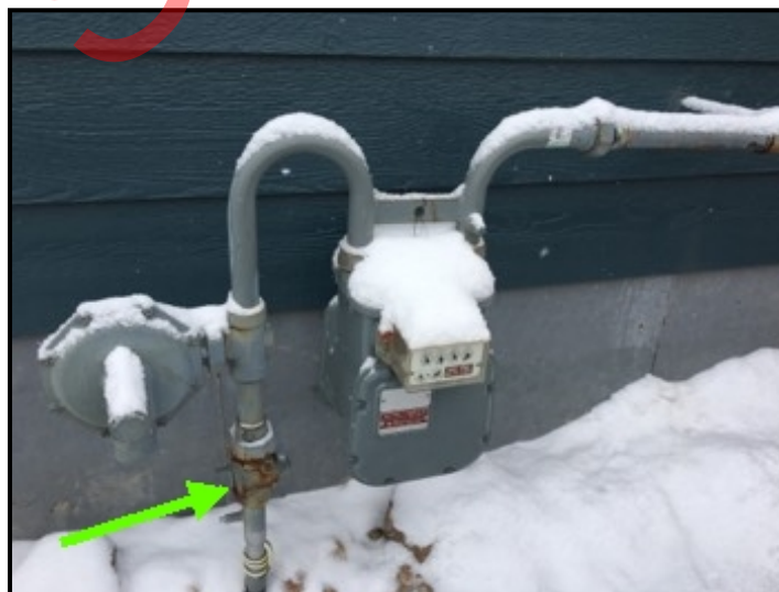
Gas meter and main gas supply shut off valve for the home.
