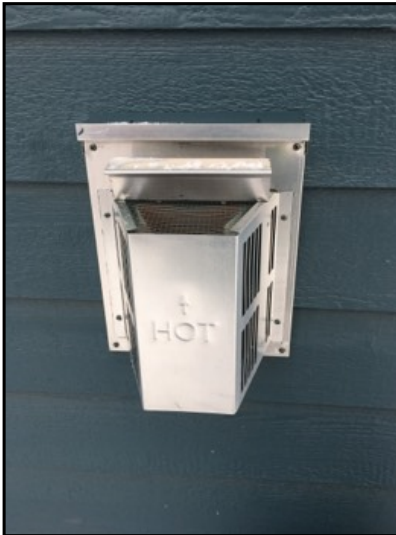
Fireplace gas flue appears functional.
