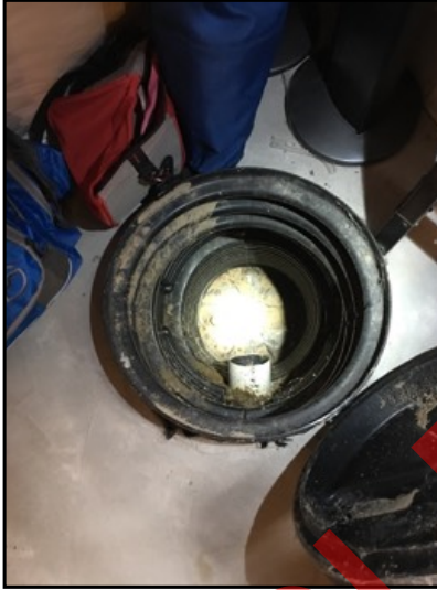
Pit is dry with no signs of water.
