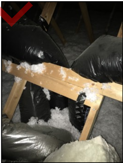
The ducts in the attic are very nicely wrapped.
