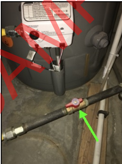
Gas supply shutoff valve for the water heater.
