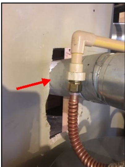
No double wall pipe through penetration as required.
