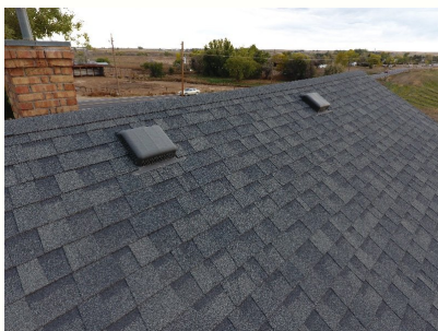
ridge vents in roofline.
