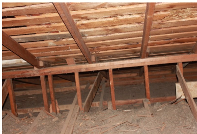
Attic roof sheathing and rafters.
