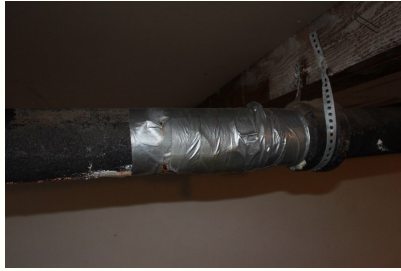
This pipe appears to have an improper repair to it, and is not properly supported.
