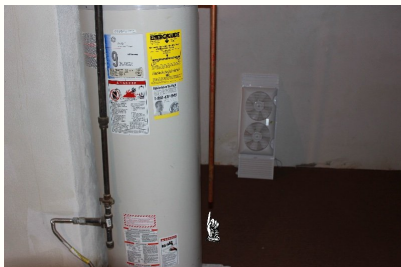
Improper termination of TPR relief valve drain pipe.
