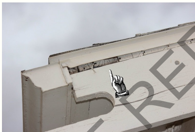
Improperly installed flashing, the flashing length is not sufficient to cover the gap, thus allowing water penetration.
