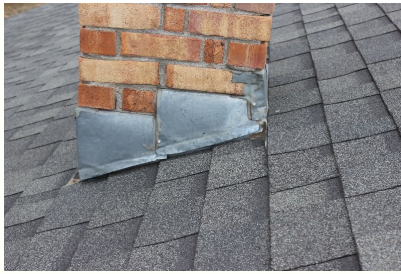
Improperly installed step flashing.
