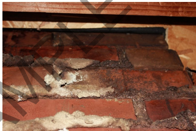
mortar joints on chimney stack in the attic showing deterioration. efflorescence is also present indicating past water damage.
