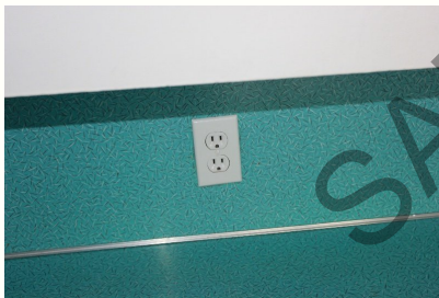
Non GFCI outlet in the kitchen.
