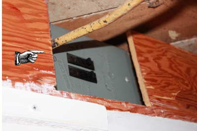
This sub-panel located in the basement rafters is not in a proper location.
