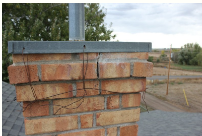
Rain cap improperly secured to chimney. Mortar failure and cracking in the brick joints.
