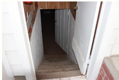
Basement access door from the backyard improperly opens over the stairs. This is a safety hazard and the door needs to be reversed to swing outwards. The door is not designed for exterior use and thus is deteriorating and should be replaced at the same time.
