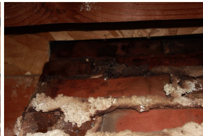
Brick chimney stack in attic showing improper repair to deteriorating mortar joints.
