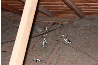
Antiquated knob and tube wiring improperly installed. This is a serious concern and should be examined and upgraded by a licensed electrician as soon as possible.
