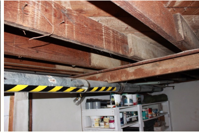
These sections of the drain waste pipe appear to have been improperly repaired with sheet metal duct pipes and sealant.
