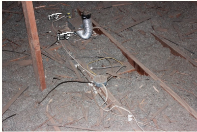
Improper termination of bathroom fan, wiring splice is not properly contained in an approved covered box.
