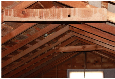
Roof frame showing OSB sheathing over former roof battens, supported by 2"x6" roof rafters. Two collar beams can also be seen adding support to the rafters.
