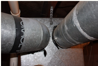
The sealant tape is begging to pull loose from the joints around the furnace and ductwork.
