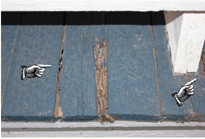
Wood deterioration on front porch decking.
