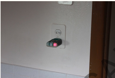
Electrical outlet showing a bad ground on outlet tester, also needs to be upgraded to GFCI outlet.
