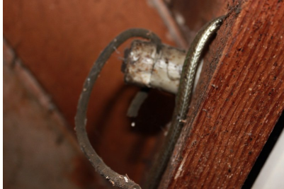
What appears to be abandoned Knob & Tube wiring in the basement rafters.
