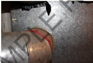
The red tape in this picture is not of the type typically used to seal duct joints.
