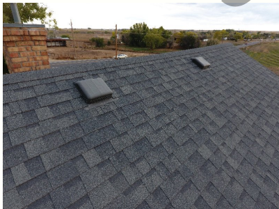
roof shingles and vents on the south back side of the home.
