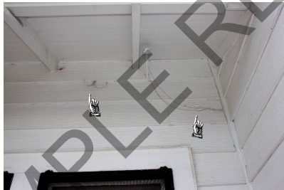
Wiring not properly installed within an approved box with cover, and abandoned wires.
