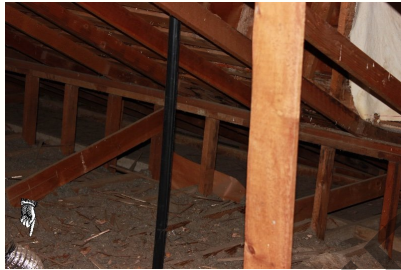
Improper termination of bathroom vent in attic.
