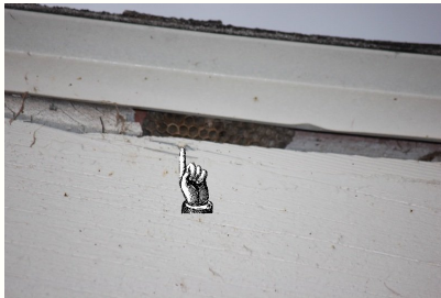
Evidence of wasp infestation in the eave rake on the north east front of the home.
