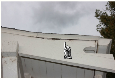
Flashing should properly extend over this gap and sufficiently onto the 2"x8" outer roof rafter below it.
