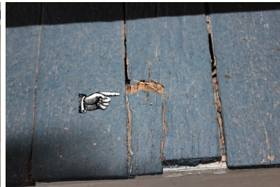
Wood deterioration on front porch.
