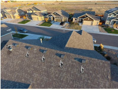
Drone picture of roof, fingers pointing at the ridge vents for the attic.
