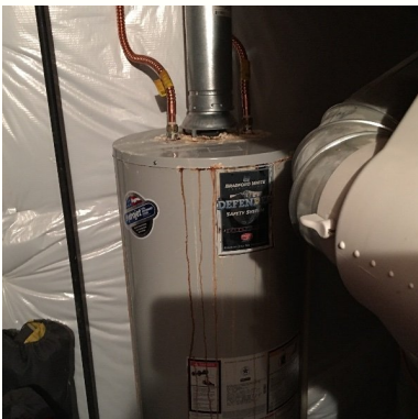
Hot water tank showing signs of past leak and rust.. Heavy mineral buildup / efflorescence can be observed on the top and in the pan below.
