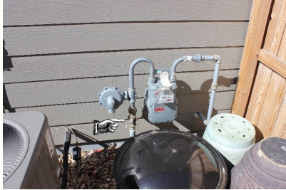
Gas meter, the finger points to the main shut off for the house.
