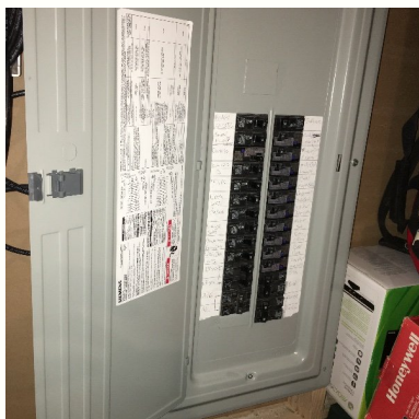
Sub panel with all circuits labeled.
