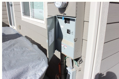
This main panel door does not properly open without removing the hot tub cover.
