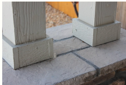
The base of these columns should be caulked to prevent water penetration.
