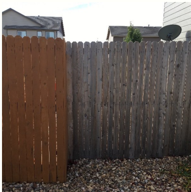
The neighbors fence can be seen on the left with a good coat of stain on it. This will help the fence last much longer.
