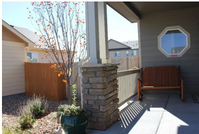
Front porch showing concrete deck, stone / wood column, and wood railing.
