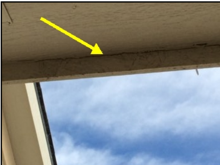
Some paint and caulk routine maintenance is needed here.
