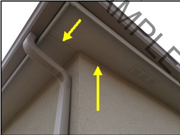
I would recommend keeping these soffit joints sealed / caulked.
