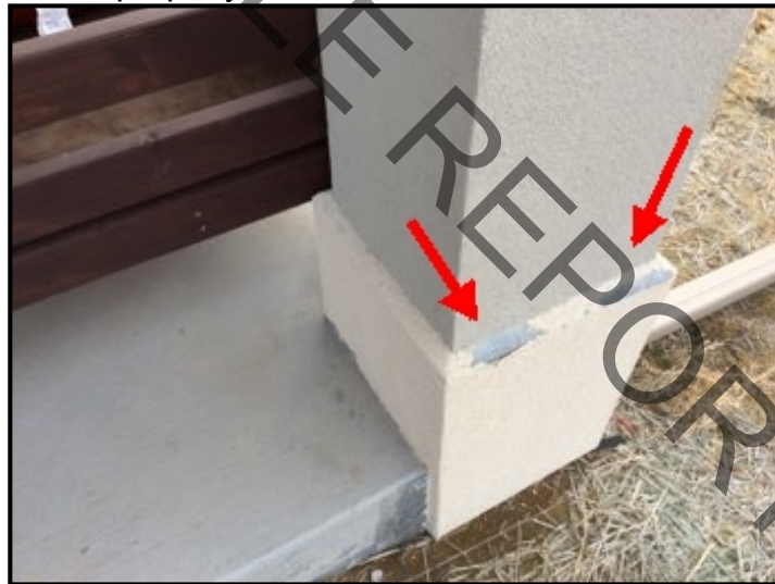
I would recommend touching up the paint in areas like this.
