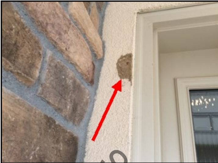
This area of Stucco at the front door appears to have been repaired improperly.
