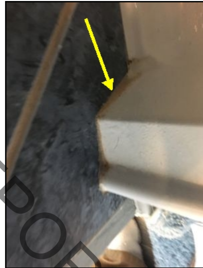
A small pocket of mildew can be seen here on the other side of the door as well.
