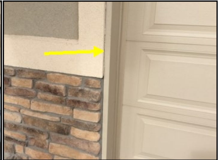
Again the joint between the stucco and trim should be caulked and maintained annually.
