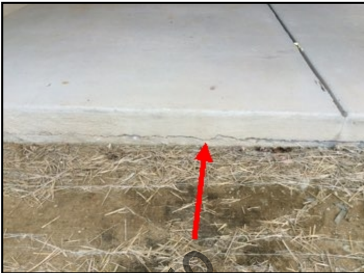
West side of the back concrete patio shows the same crack extending fully around two sides.
