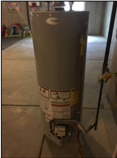
TPR valve is correctly installed and plumbed to the floor drain.
