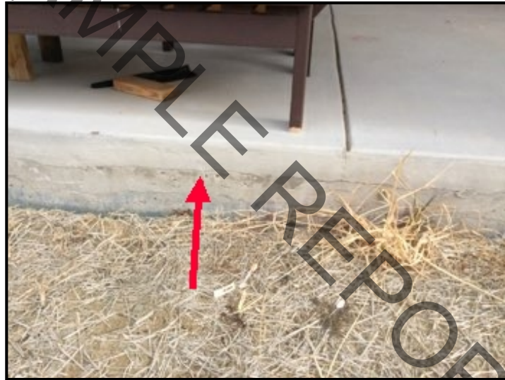
Continuation of the crack on the west side.
