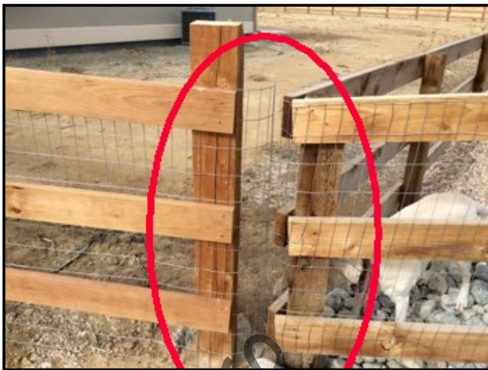
The fence is not properly tied into the neighbors corner.
