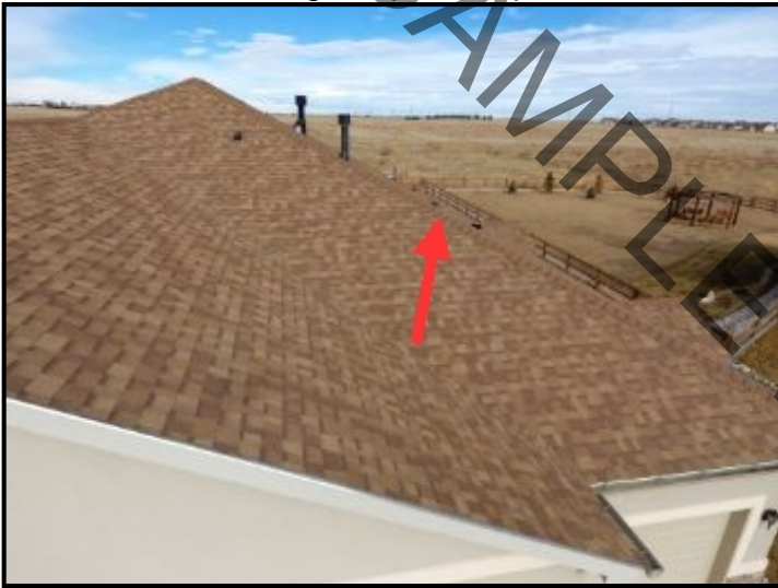
Roof valley and ridge, this ridge is wavy.
