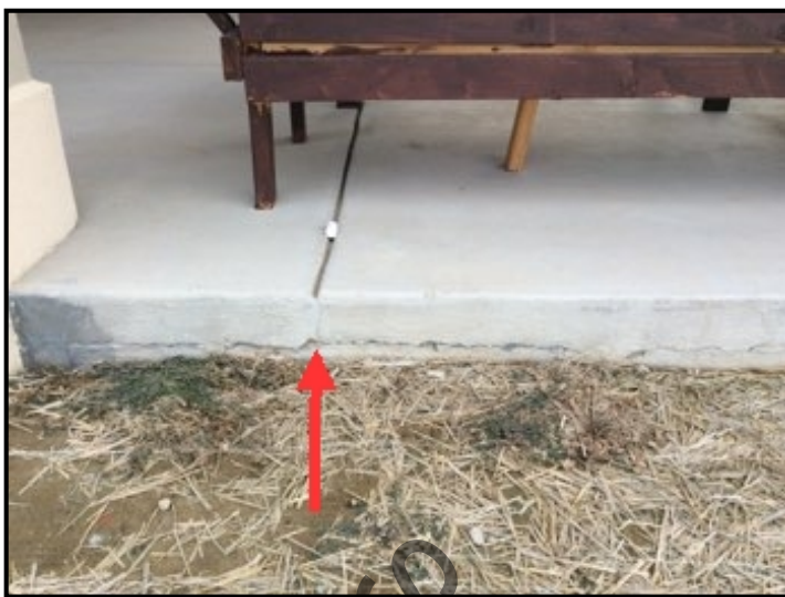
North side of the back patio. This crack is of some concern, a similar one is starting on the front concrete porch as well.
