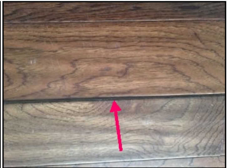
Gap in floor joint.
