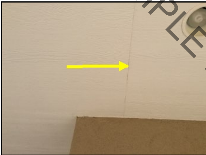
This joint could use a little caulking on the ceiling of the covered patio.
