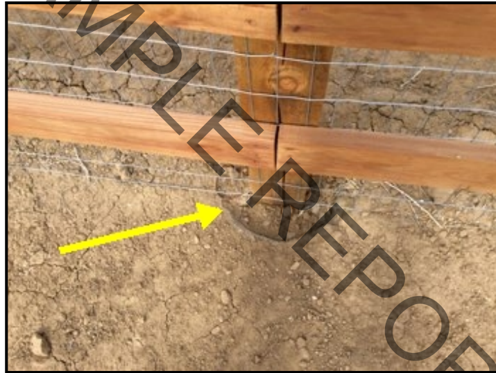
The concrete around the post was not installed very well and creates a bowl to hold water. This will accelerate water damage / rot to the post.
