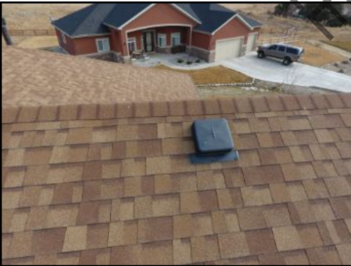
Attic turtle vent properly installed.
