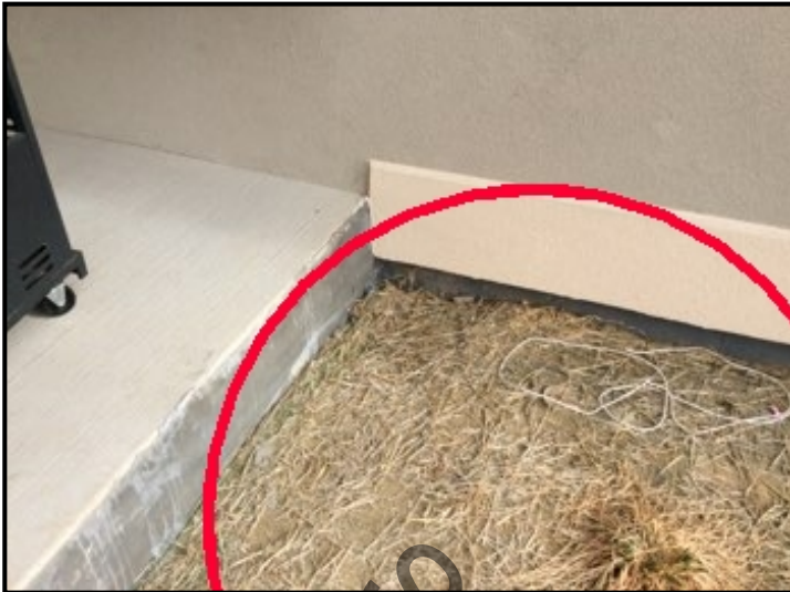
This area is slightly low and may hold water, when the landscaping is completed grading should promote a slope away from the foundation of 6" within the first 10'
