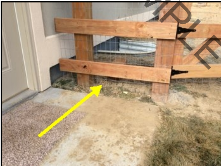
This area by the east gate is draining onto the stoop and will eventually cause problems here. Special attention should be taken when landscaping is complete to promote drainage away from the house but not over the concrete pad.
