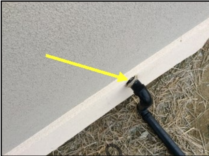
The sump pump drainage pipe needs resealed where it exits the house.
