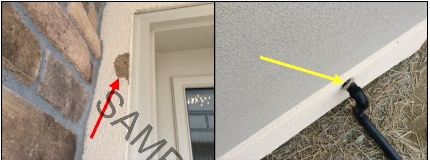
This area of Stucco at the front door appears to have been repaired improperly.
