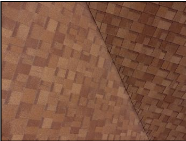
Covered valley on roof properly over lapped.
