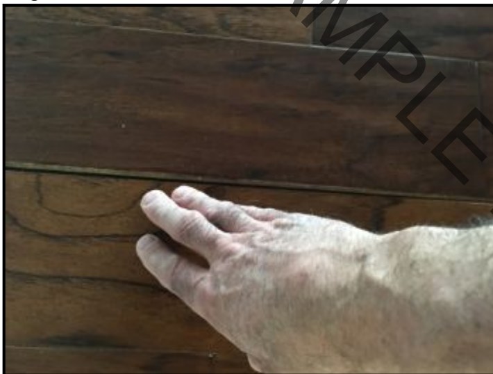
Gap in floor creates flex / bounce on adjacent board.
