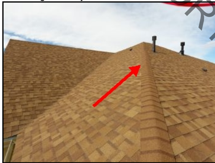
This roof hip is wavy in appearance.
