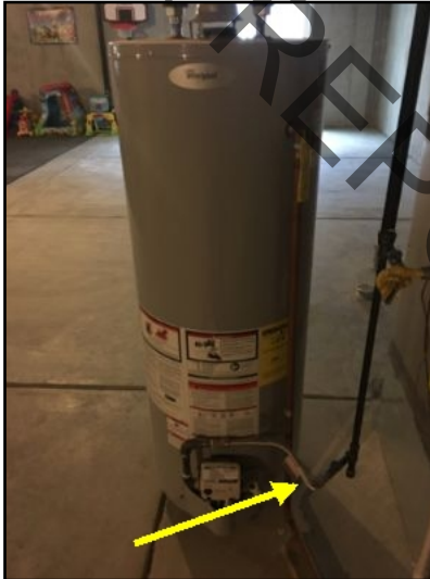
The water heater appears in good condition. Gas feed shut off is located at yellow arrow.
