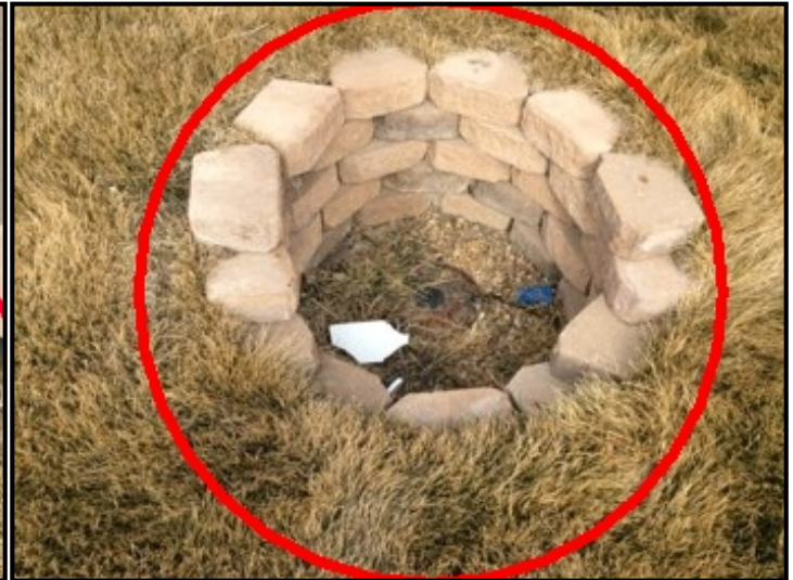
This meter is a safety hazard and should be repaired by a professional contractor as soon as possible. The meter can be raised with a sleeve and dirt filled in around it, there is no reason to have a trip, fall hazard such as this.
