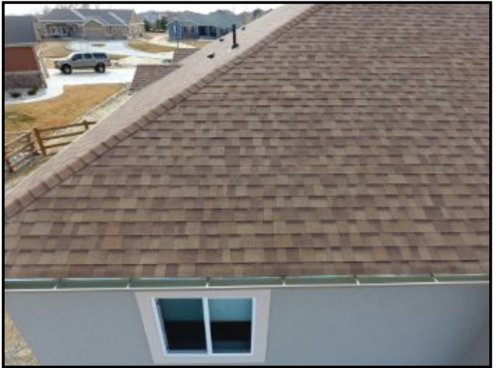
Aerial of hip and shingles on roof
