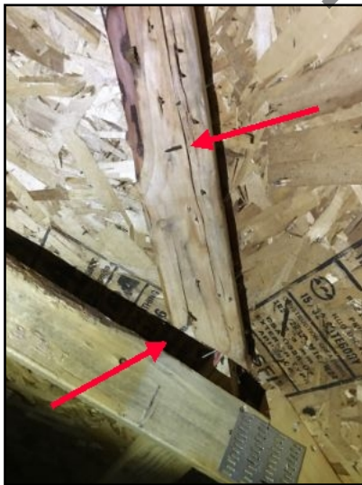
There is some poor framing and cracked lumber used in the attic for the hip support
