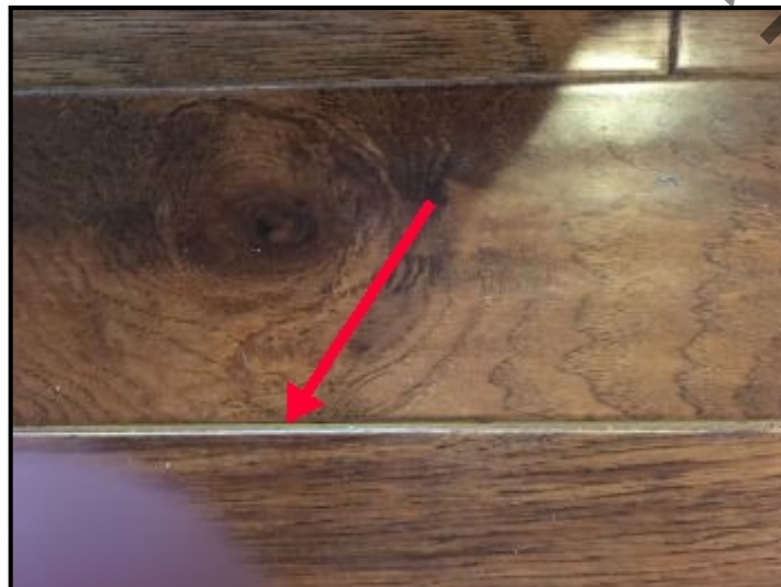
Another gap in the floor board joint.
