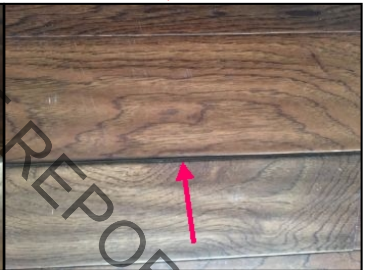
Gap in floor joint.
