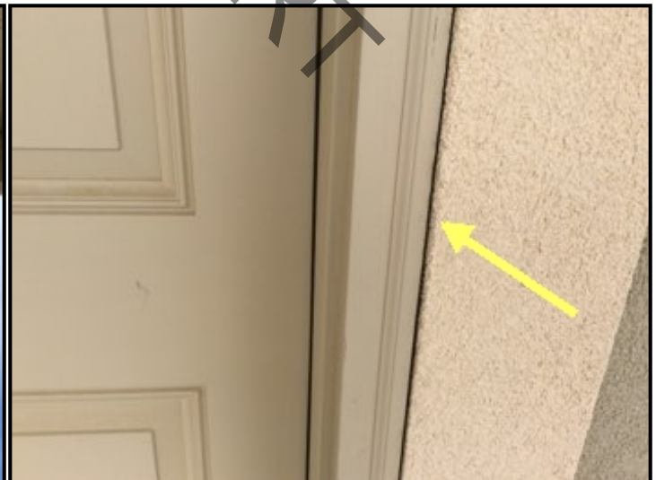
I would recommend these areas between the trim / door jamb in this photo are kept caulked and sealed to prevent excessive moisture intrusion.
