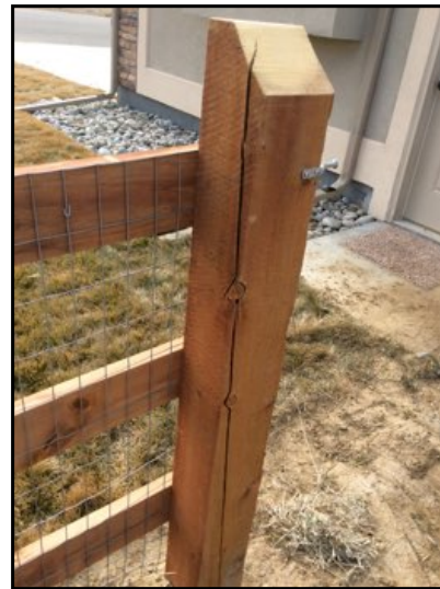
This gate post on the east gate is almost cracked all the way through and should be replaced. It is also cracked on the other side.
