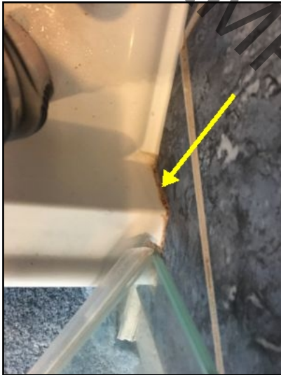
Some mildew can be seen in this corner and should be easily cleaned out.
